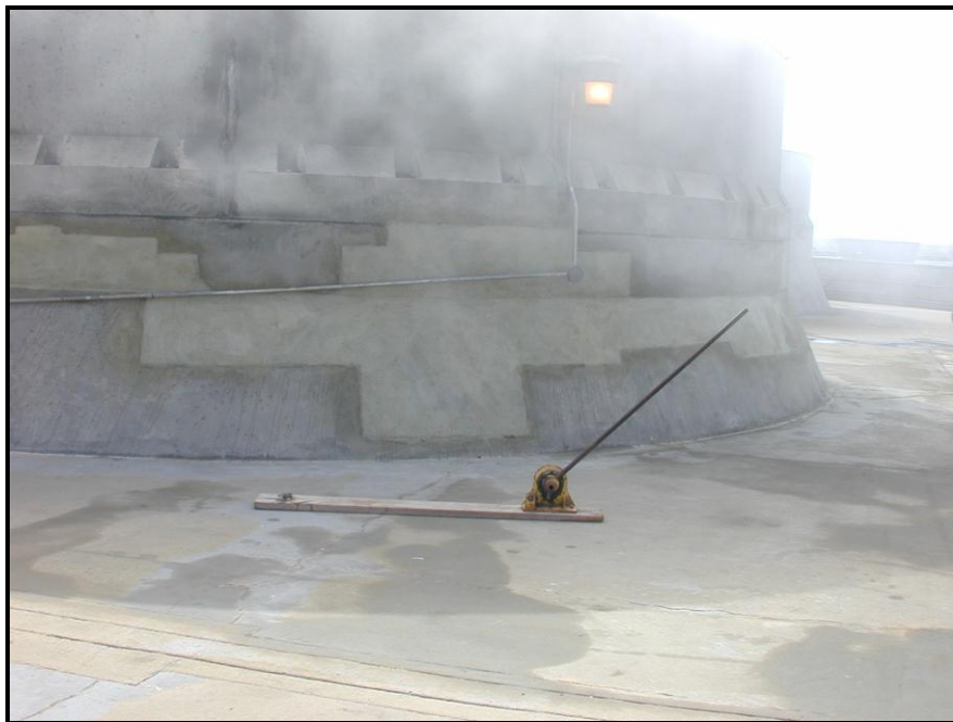
Figure 4. Completed Spall Repair at Lower Assembly
