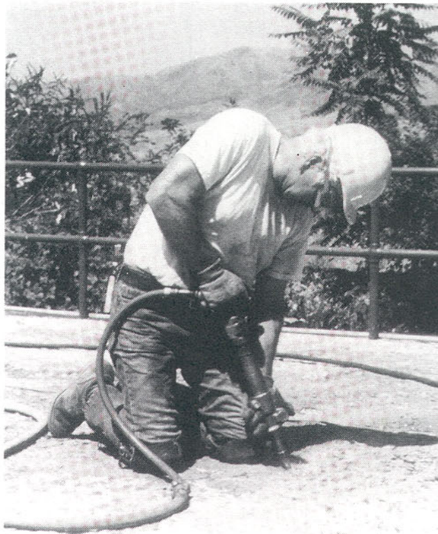
Technician prepares surface for partial depth repair with 15 lb. chipping hammer
